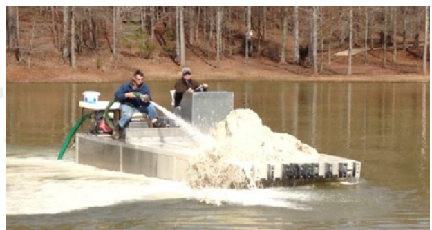
Bulk lime is applied by washing it directly into the water in such a way that it covers most of the lake bottom.
